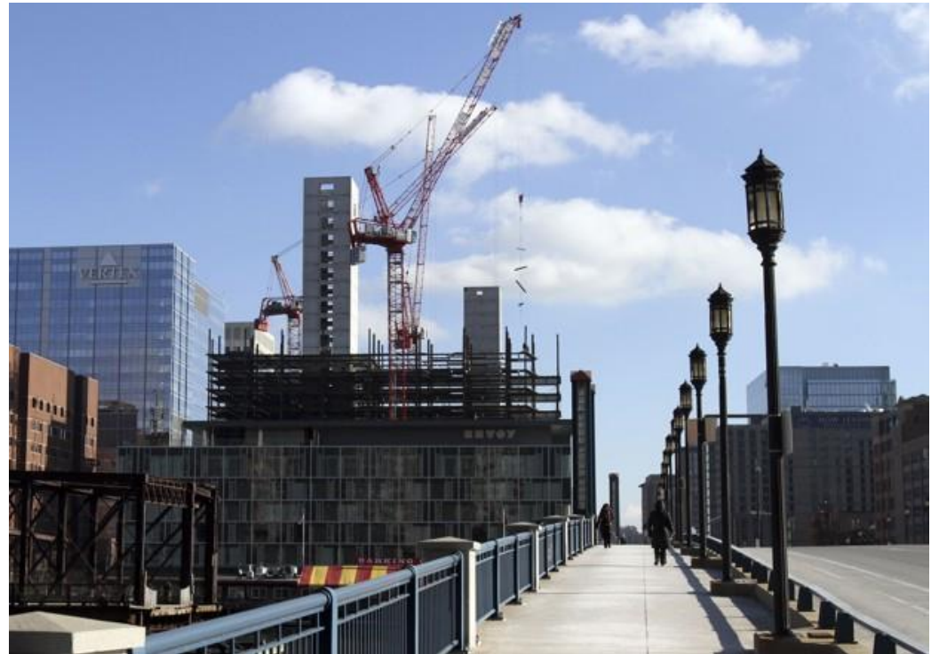
Construction in Boston's Seaport Neighborhood
