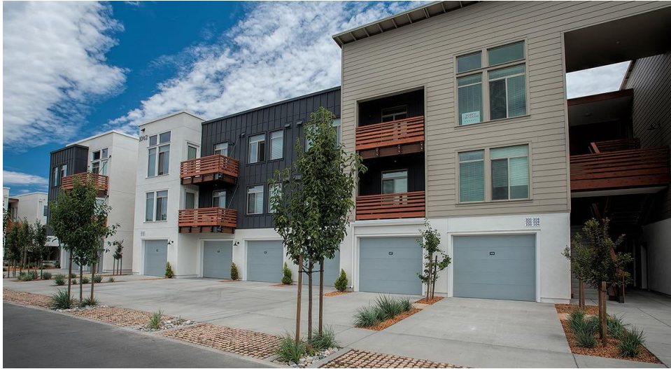
Annadel Apartments – Kattera
