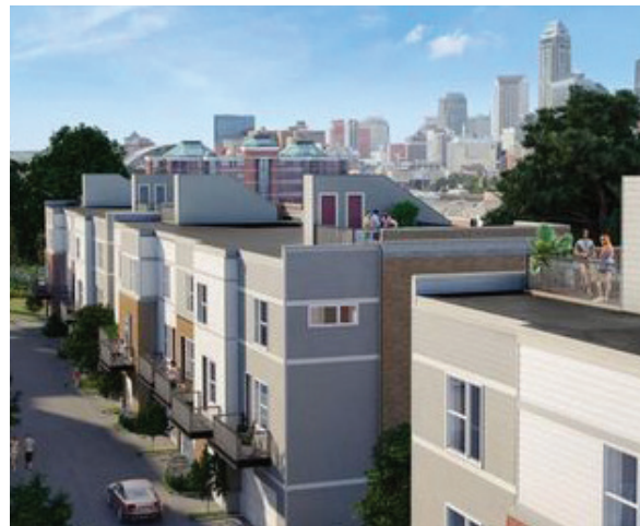
Onyx & East, Switchyard at Fletcher Place, Indianapolis. (Onyx & East)
